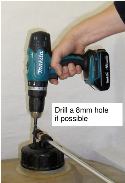
Measuring pipe mounted in tank ventilation
